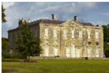
The West Front at Claydon
