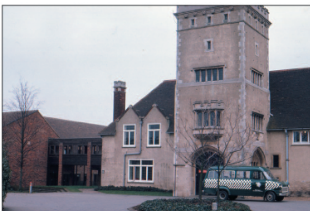
The headquarters of Milton Keynes Development Corporation, Wavendon Tower
