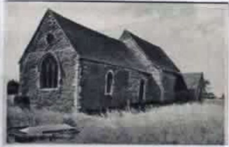
St Peter's Church Stanton Low - The original Norman church serving the manor of Stantonbury until 1860. Sadly, now a ruin.
