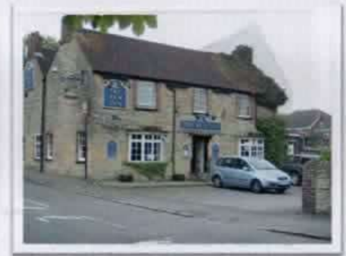
The Wharf Inn – the oldest building in new Bradwell, built in 1804. Now known as the New Inn.
