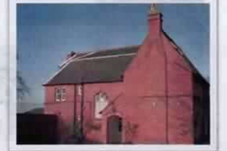
The Vicarage situated on Bradwell Road was designed by George E. Street and built in 1858
