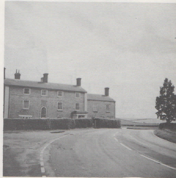
2. The Manor House, (grade 3)
