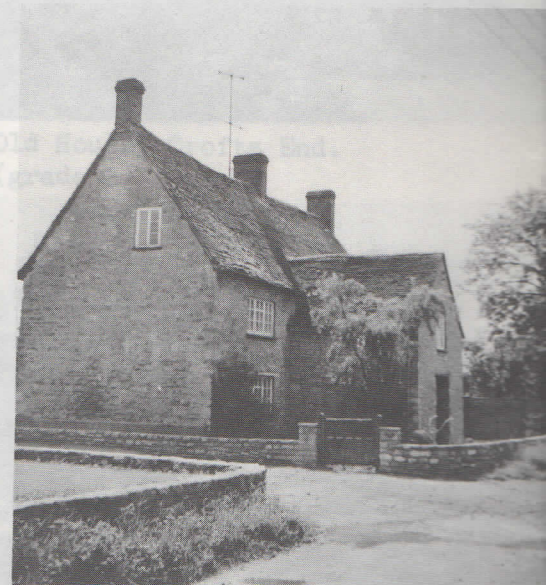
12. Water Lane Farmhouse (grade 3)
