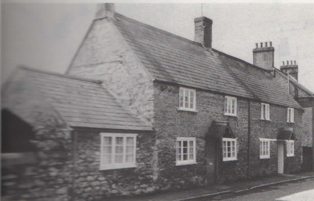
18C cottages, Crofts End, (grade 3)
