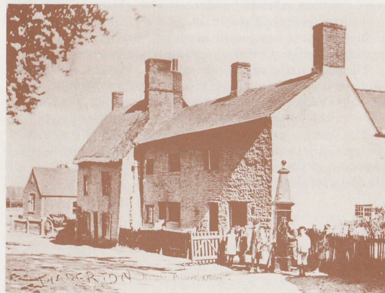
Water pump Emberton
