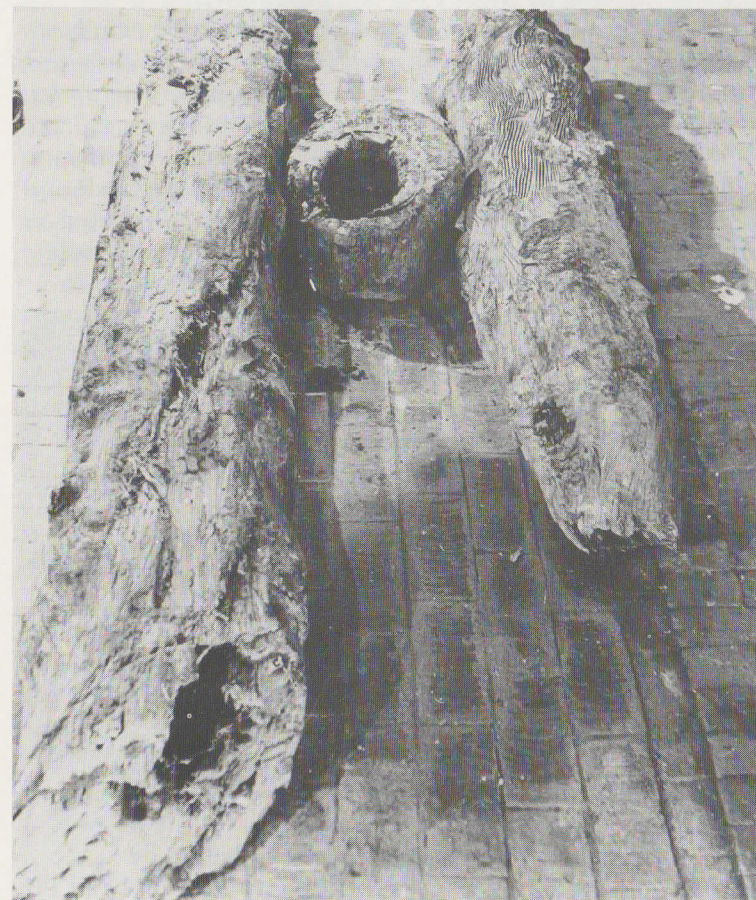
Water main from Newport Pagnell High Street
