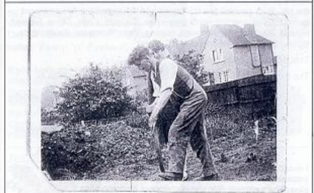
SID TATHAM, DIGGING THE FOOTINGS FOR THE VILLAGE HALL C 1920'S
